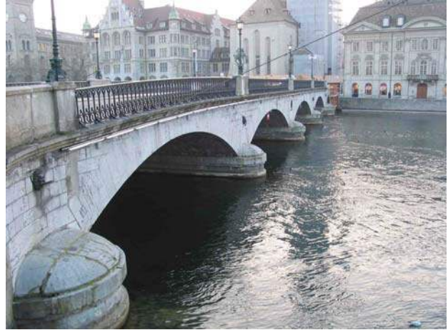
b) Road bridge in Zurich
