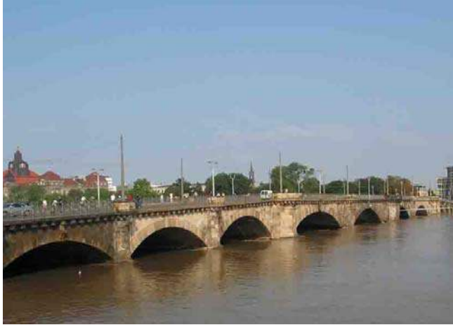
a) Albertbrücke in Dresden at high water mark
